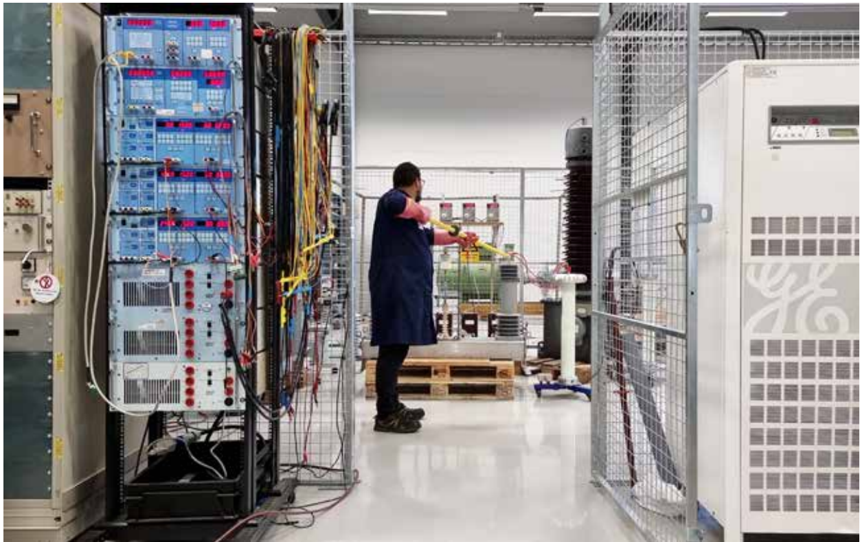
Testing of a switch in electric medium voltage test cell
